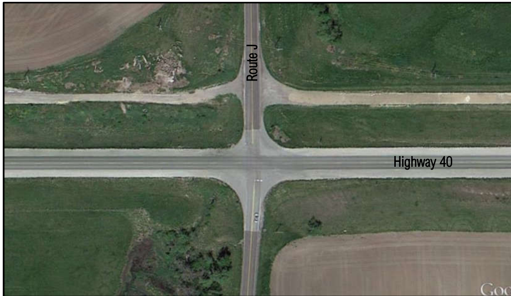
Figure 4: Highway 40 and Route J Intersection
