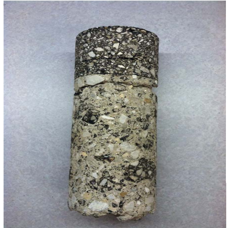
Core from Gibbs FDR project after completion. Displays sturdiness of rehabilitated base and strength of bond between asphalt & base
